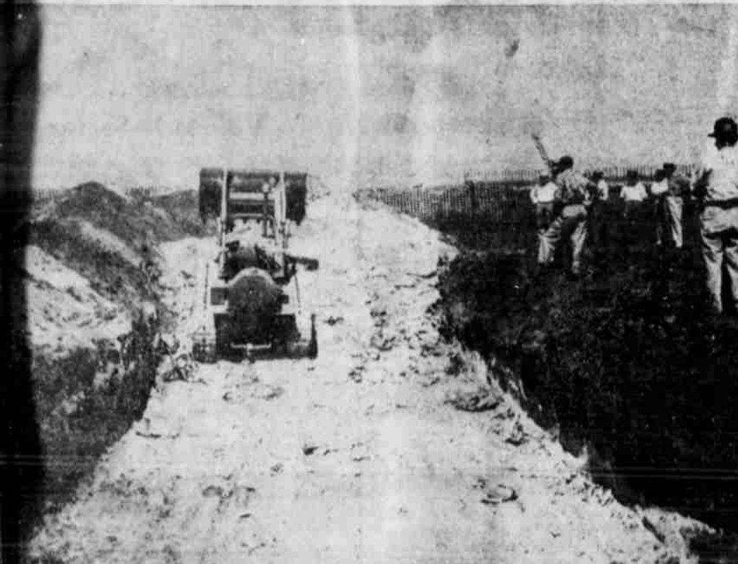
Garbage disposal by the sanitary landfill method is illustrated above. The trench above, 17 feet in depth averaging 5 feet in depth, was filled with trash and refuse before the operator began digging and covering it. The garbage is buried at one end of the trench and sealed with cover material dug from the other end of the trench. At one end of the trench is filled with cells of the other end will be extended to the end of the city property. When this trench is completely filled and covered, another trench will be dug parallel to it. Garbage will now be picked up from the residential sections twice weekly and will be collected daily in the business district. (Photos by Taylor Studio)
