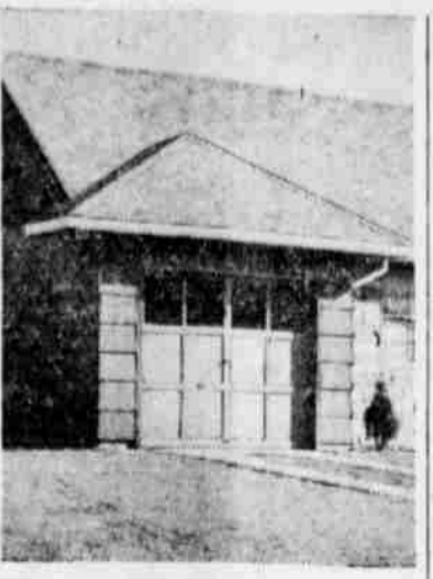
This garage is under the same roof as the house, but a hip roof- style projection over the garage adds variety to the design. Asphalt shingles are blended.
