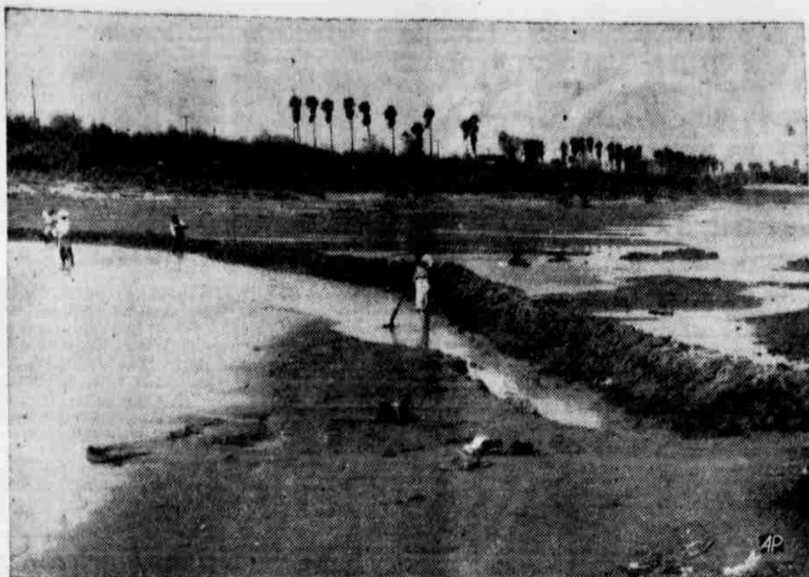
Farmers of the arid vegetable growing area south of Brownsville, Texas, have protested against this earthen dam constructed across the Rio Grande
