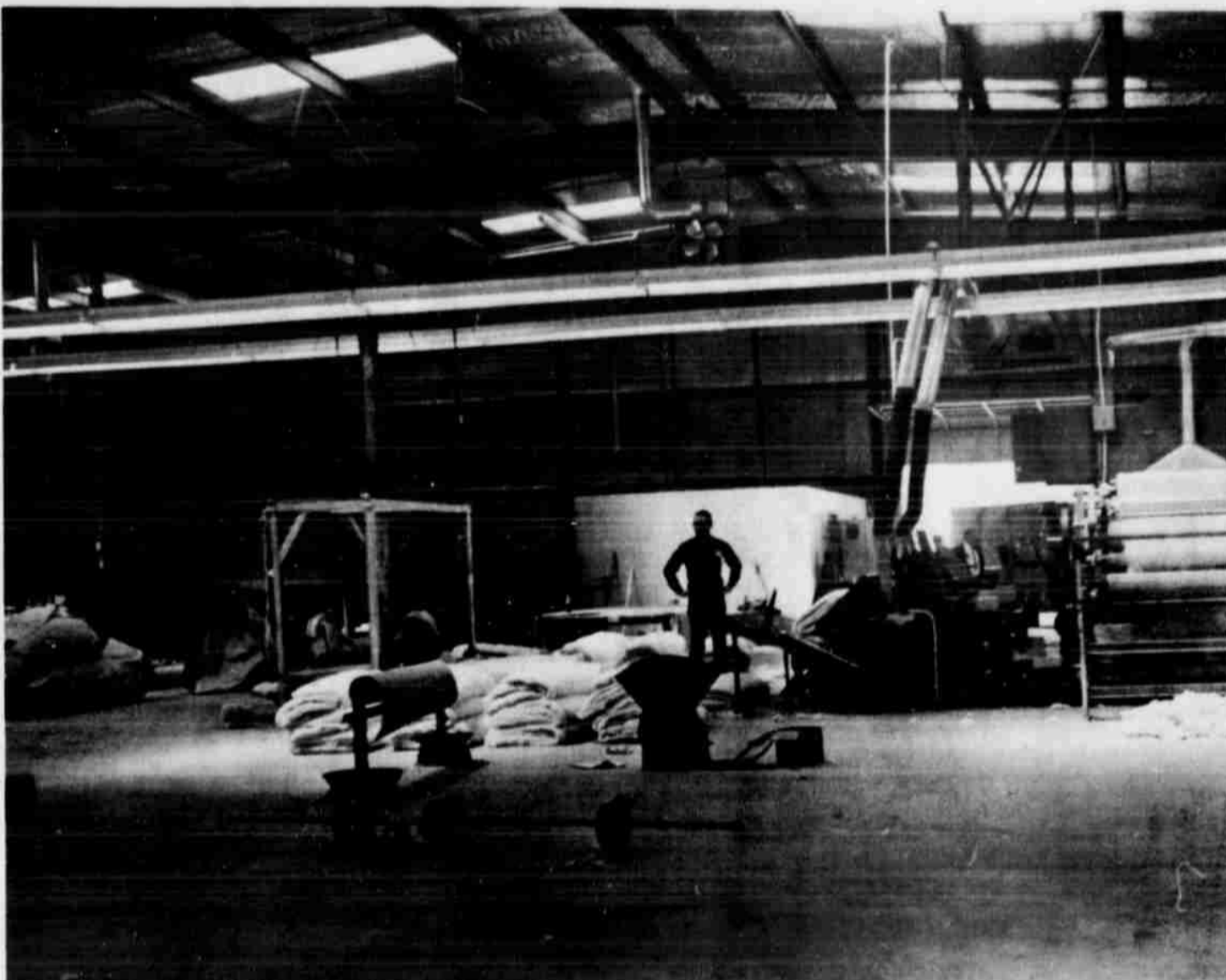
WORK UNDERWAY -- A depth shot of the plant shows Ronny Smith standing among cotton bats ready for baling. In foreground device on wheel-type mounting feeds paper dividers between layers of bats. Plant Manager Bill Damron explained
