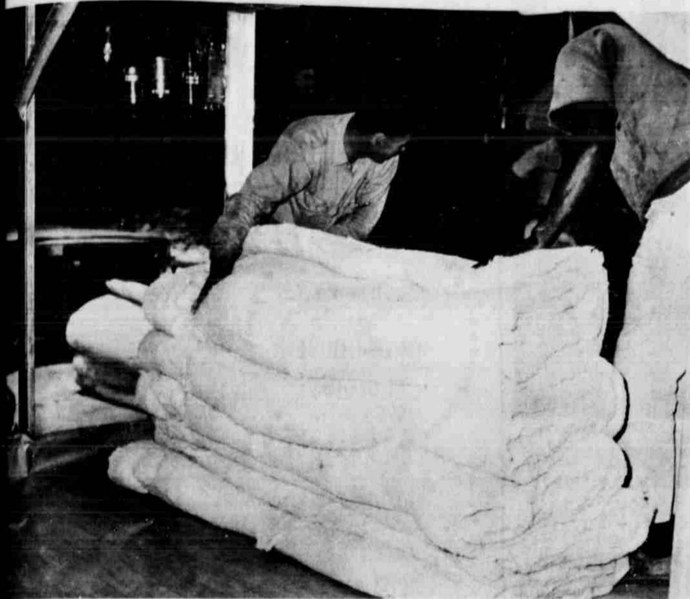
WORKING PRESS -- Finished cotton batting is placed on baling press by employees. Note portion of press shown at top of photo. When filled the press will lower and compress the batting into
