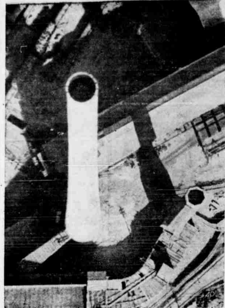
SMOKE'S EYE VIEW—This aerial view taken from a plane 650 feet above the ground shows the 611-foot, 8-inch smokestack at the American Smelter and Refining Co. in El Paso, said to be the world's highest. The shadow of a nearby 225-foot stack can be seen in the picture.
