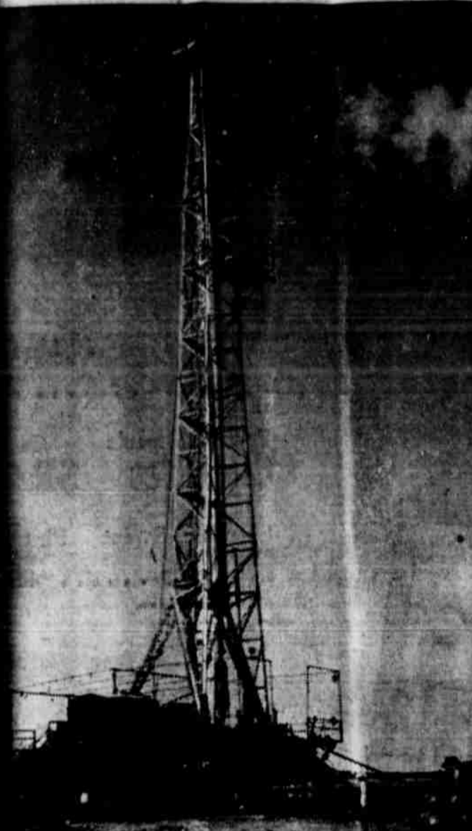
The Jack Knife Derrick, 38 feet high, and was erected on the site Sunday on the water tower on Compress property for the drilling of the first deep test to be drilled in the Littlefield townsite. Drilling started Monday morning with the tool pusher and 15 men on the job.
