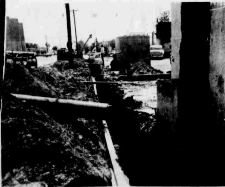
DITCHES WERE DUG AND NEW PIPES WERE LAID
