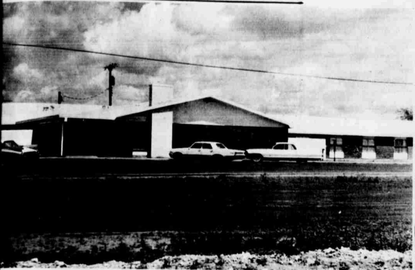
SETTING FOR NEAR FUTURE -- The formal opening ceremonies for the Hospitality House will be held in the near future. Located just southwest of Littlefield, the convalescent home will house a maximum of 50 persons and will incorporate many new ideas. Built at a cost of approximately $150,000, the sprawling 14,000 square foot ranch type building will front on the Bula Highway.
