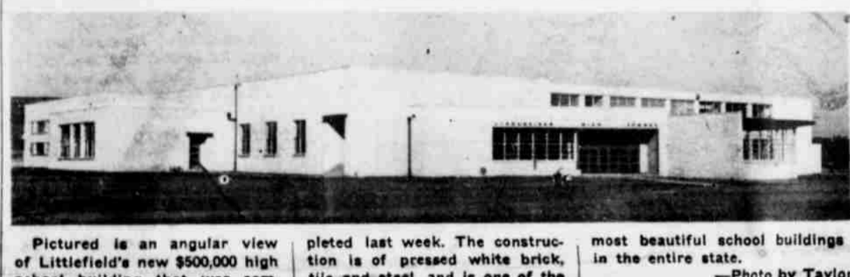
Pictured is an angular view of Littlefield's new $500,000 high school building that was com- pleted last week. The construc- tion is of pressed white brick, tile and steel, and is one of the most beautiful school buildings in the entire state. —Photo by Taylor
