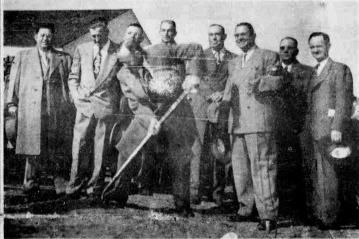
BREAKS GROUND FOR NEW SCHOOL—Mancil Hall, president of the board of trustees of Littlefield Independent School District, is pictured above turning the first spade of dirt as construction of a new $500,000 high school building started here Monday. Gathered around Hall are other school trustees, officials, and the building contractor. Left to right are Jack Yarbrough, trustee; Boyd Montgomery, trustee; G. G. Wilson, trustee; A. D. Gistrop, contractor; Carl Arnold, school secretary; Jack Christian, trustee; W. O. Hampton, trustee and Joe Hutchinson, school superintendent.
