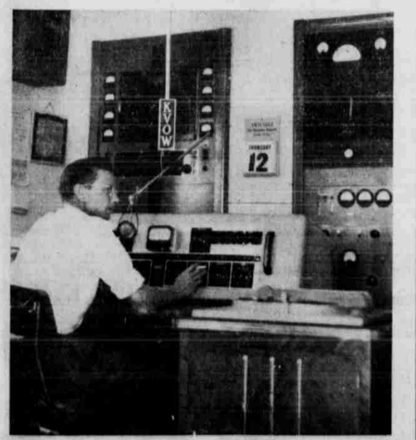
—Pictures by Taylor's Studio. Heart of Radio Station KVOW is this modern control room which regulates all the station's activities. Seated at the controls is J. W. Robinson, chief engineer.
