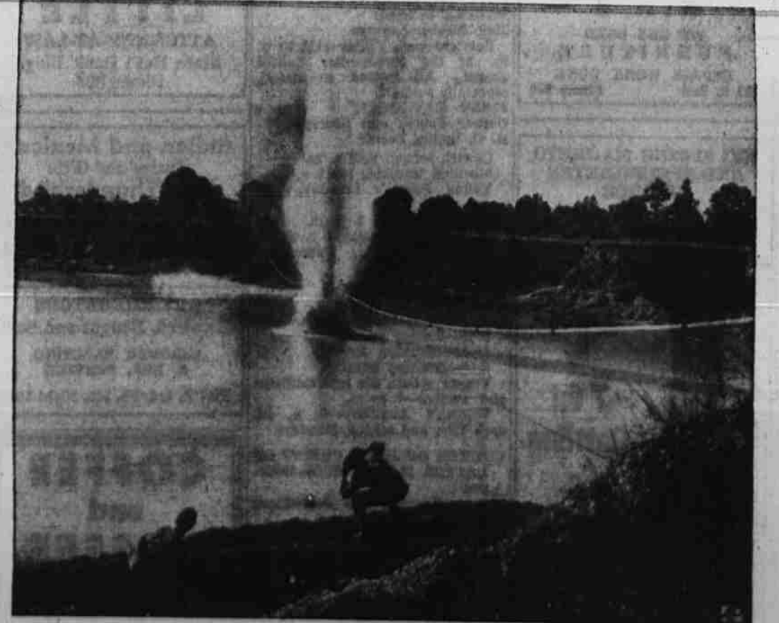
BENT BUT NOT BROKEN —A simulated bomb burst throws up a geyser of water but merely bends a portable oil pipeline built by engineers in training at Camp Claiborne, La.
