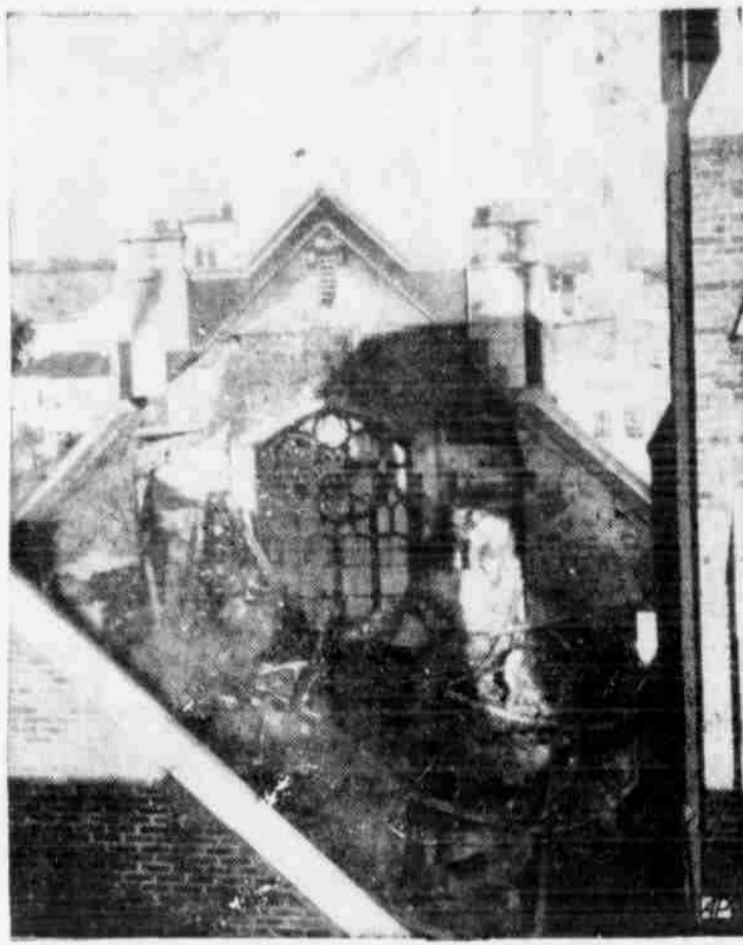
WELL-KNOWN CHURCH BURNS—The roof of the sanctuary of Waco's Austin avenue Methodist church block-long structure where thousands of Texans have attended conventions, is shown after it collapsed during a fire. (AP Photo)
