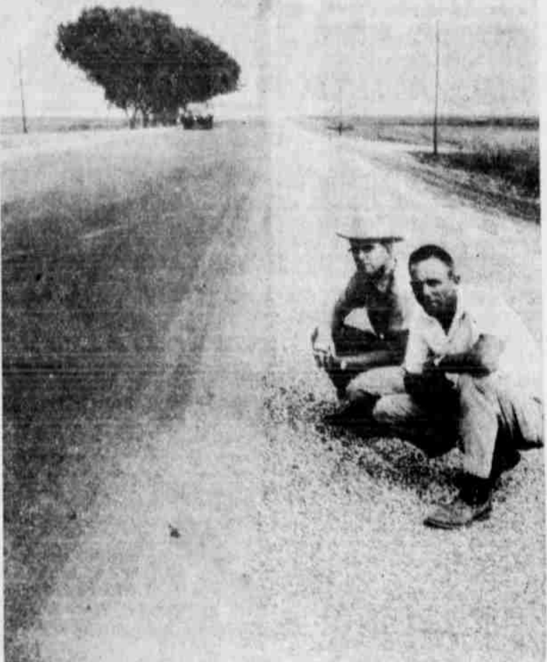
FINAL INSPECTION —Rhea Bradley, at rear, State Highway Department resident engineer, and H. C. (Doc) Brown, inspecting engineer, look over new construction on Highway 51 north of Littlefield. Work on the $450,000 project was completed Saturday. Center line will be painted this week. The new construction includes a 26-foot-asphaltic concrete roadway with eight-foot paved parking shoulder, the highest type two-lane construction used by the State. The highway was rebuilt from Littlefield to 1 1/2 miles south of Springlake, where a new roadway had been completed earlier. Contractor on the job was Henry L. Stafford of Lubbock. (STAFF PHOTO)
