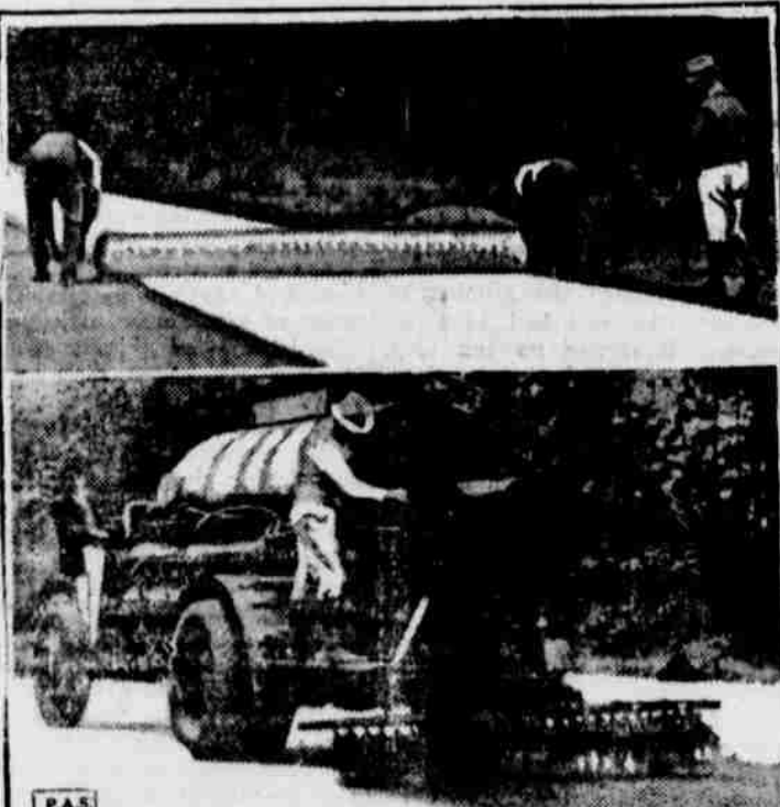
SCOTT, Miss. . . The first "Cotton Highway", a 14-mile experiment in road construction, is rapidly nearing completion here. The upper picture shows the cotton fabric membrane being rolled out on the highway on a base of mixed clay and gravel. Lower picture shows coat of tar over cotton, this covered with two applications of asphalt mixed with screen gravel.
