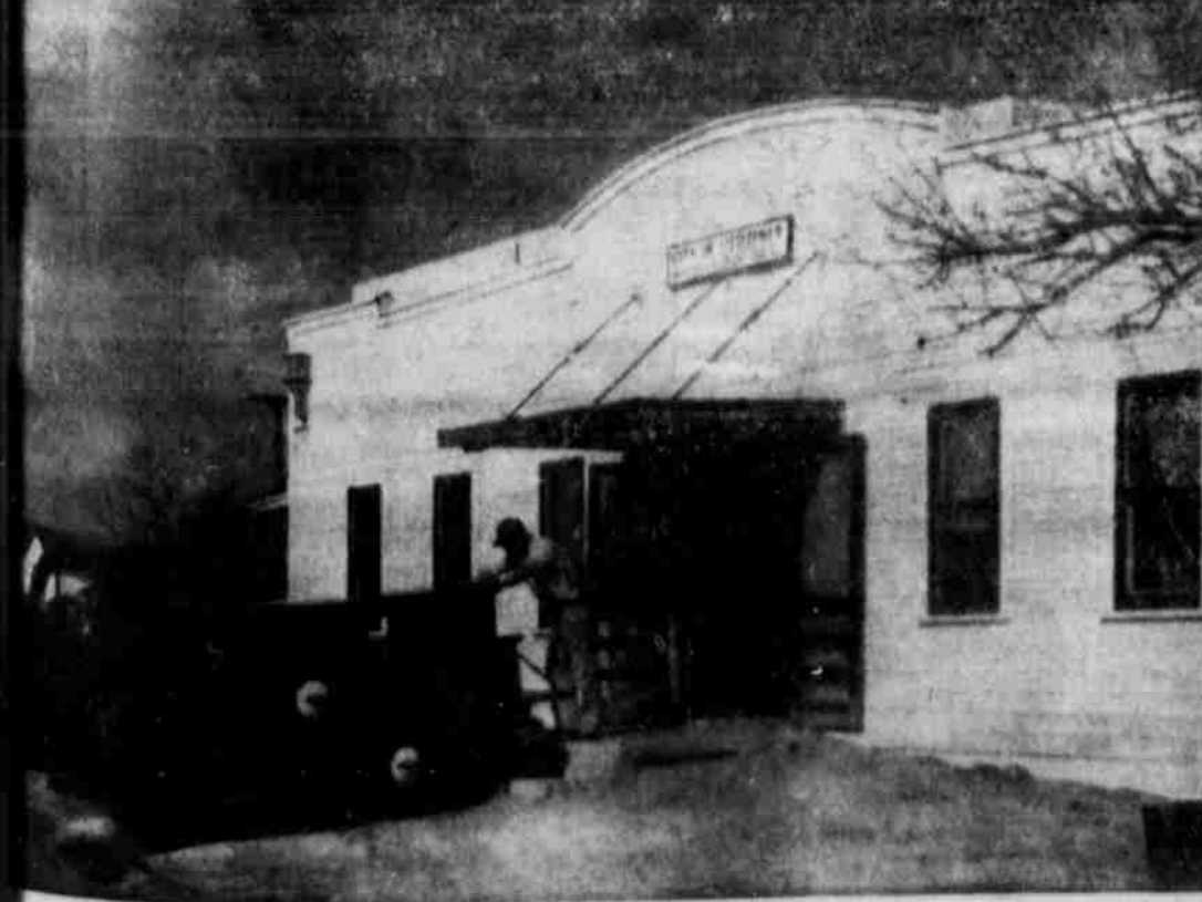
CITY OFFICES ARE BEING MOVED this week from the "temporary" location on the east side of the square where they have been for the past nine years. City officials are moving into the City Hall building facing Phelps after the building has been redecorated throughout. All city business will be transacted in the City Hall after Thursday, today.
