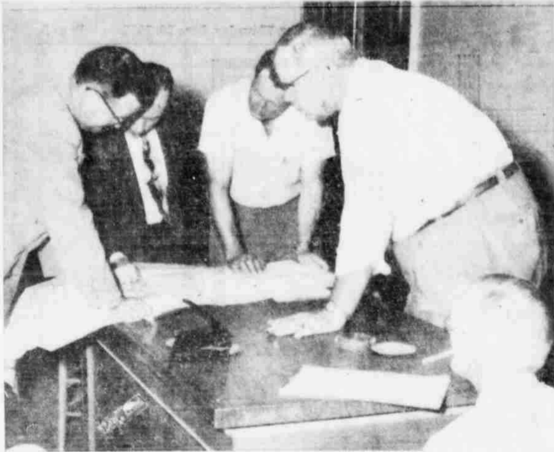
CITY SIGNS OIL WELL PERMITS. Shown looking over a map of the city, divided into drilling blocks, are members of the Littlefield City Commission and a representative of the Texas Co. Pointing out the location of the two new wells on the map is Bill Boone, Texas Co. attorney, second from left. Bill Street is at the extreme left. Commissioner James Crump and Mayor Ray Kneeling look on. Seated is City Secretary W. G. Sacket. (Staff Photo)
