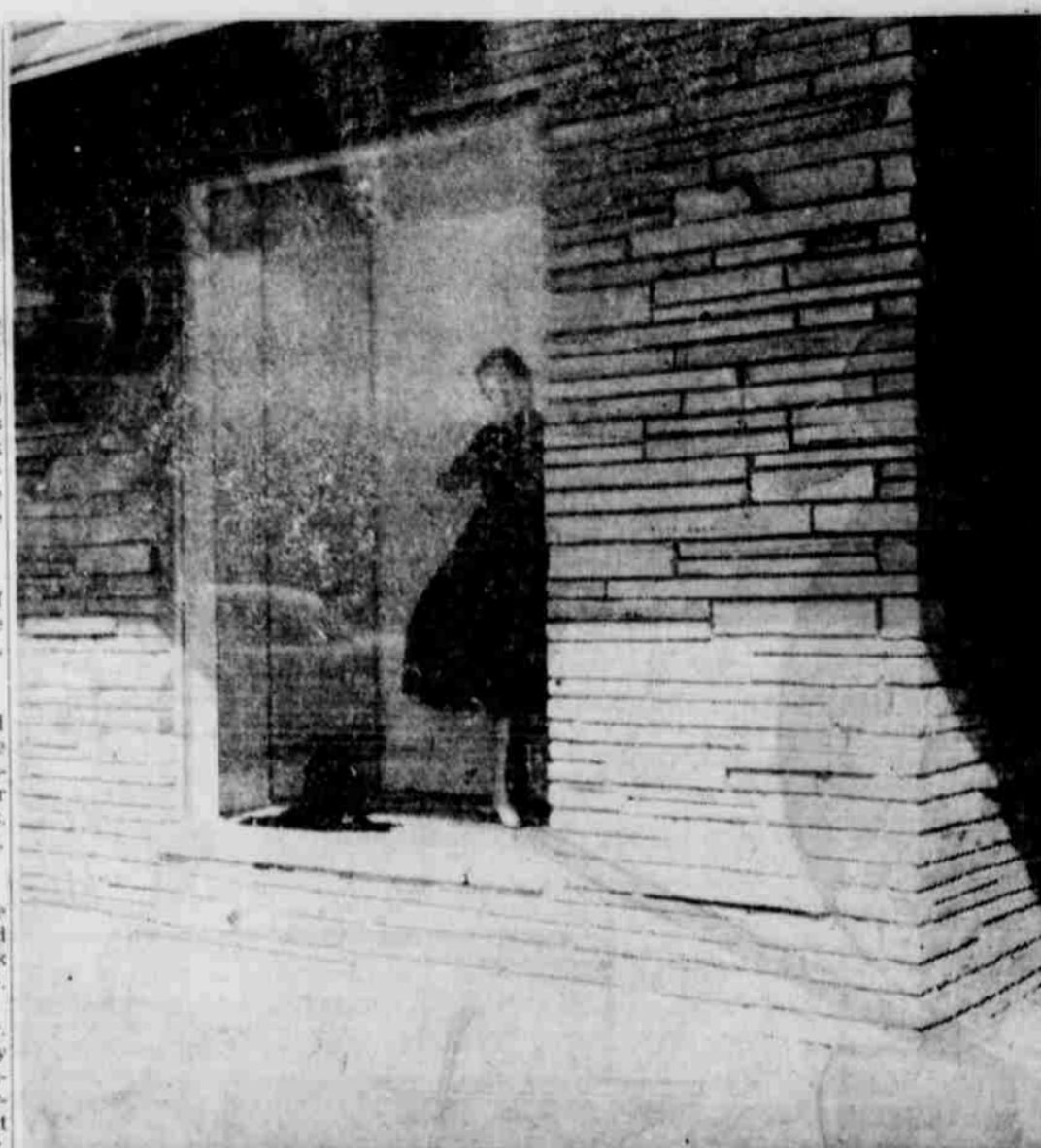
Arkansas Stone, miniature display windows are keynote of Ware's new store front.
