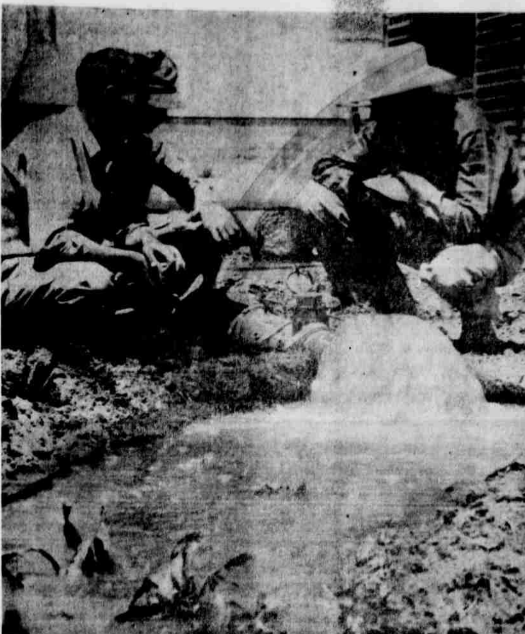
ACIDIZING WATER WELLS. Helping to improve the GPM flow of irrigation by acidizing wells can be a big boon to county farmers. Here, Jack Carrigan, an acidizing company representative, left, watches a test flow from a well belonging to Norman Emfinger, center, that has been acidized. Watching them, right, is B. T. Kisner, SCS official. Acidizing helped to improve Emfingers well by over 60 GPM.
