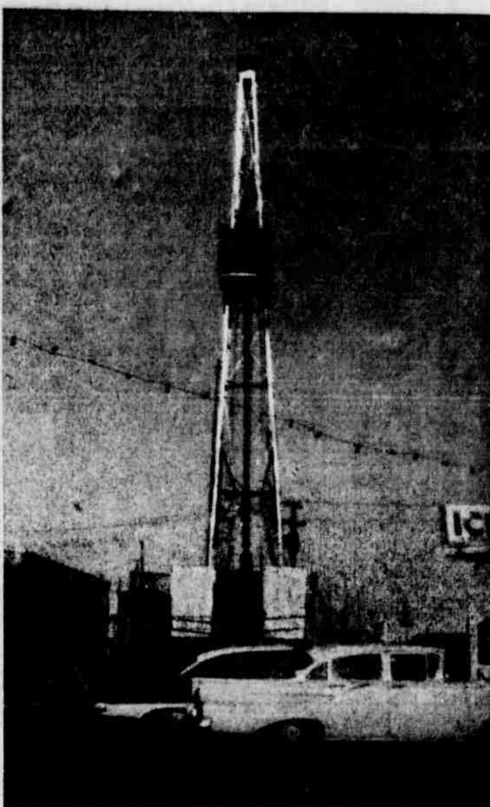
ANOTHER OIL WELL in Littlefield is being drilled just west of Renfro Bros. Grocery and had drilled down to 2800 feet Tuesday morning. It is classified as the Chesher-Pioneer oil well and is being drilled by the Sittin & Norton Drilling Company. It is scheduled to go down 4,000 ft. and should be completed around the first of the year.
