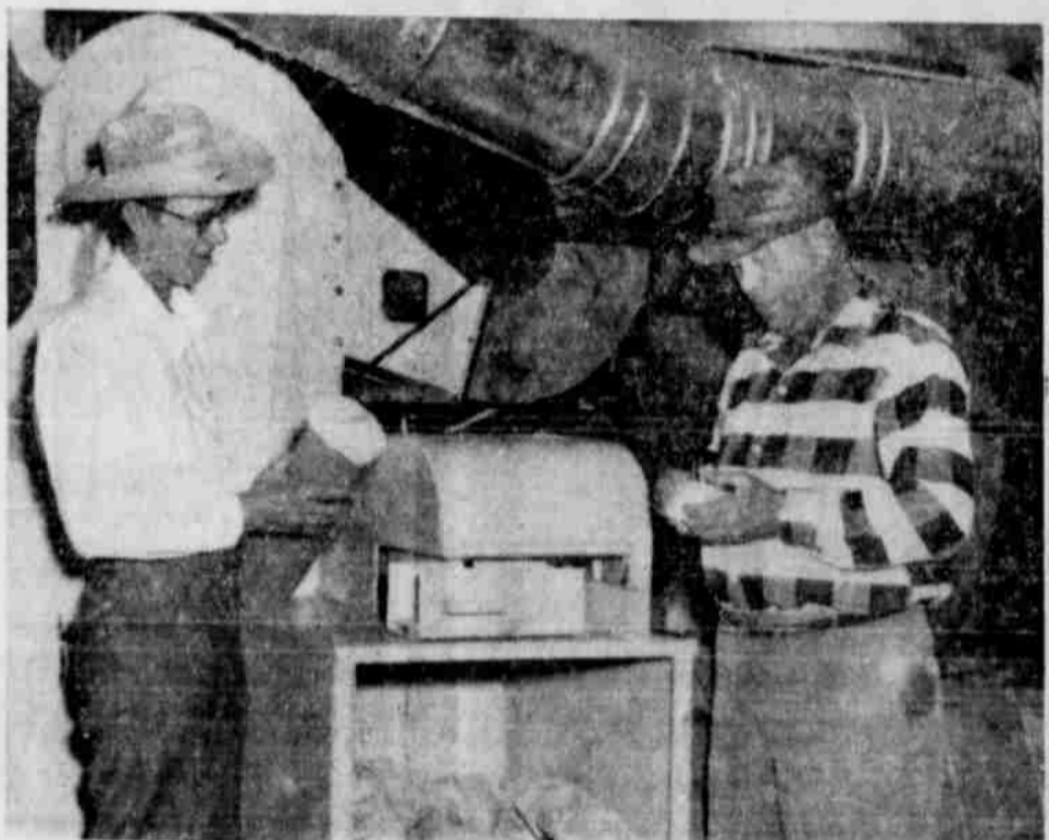
Alva Pierson and Carl Arnold look at some cotton samples from the recently installed sampler.
