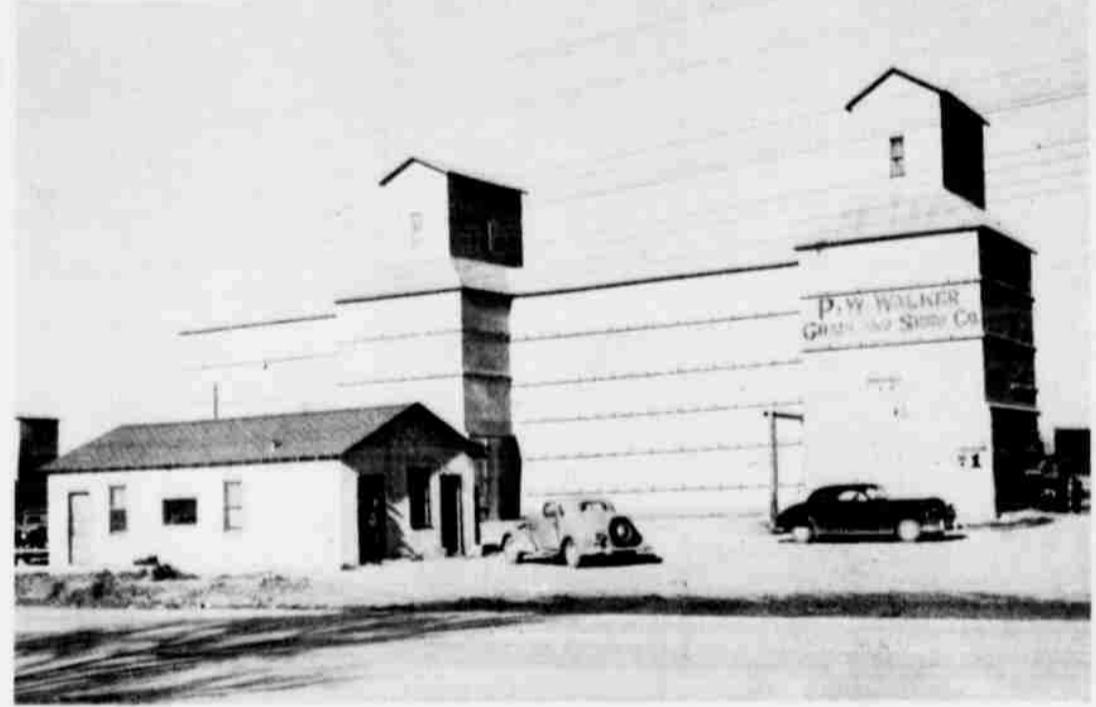
OLD ELEVATOR -- This is the P. W. Walker Grain Company which burned in 1950 after serving the people of this area for several years. Walker rebuilt the elevator and continued in its operation until last week, 33 years after he first purchased the company.
