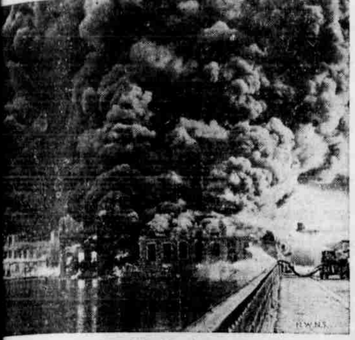
Here is a spectacular view of the fire that swept through the huge plant of the Fall River, Mass., plant of the Firestone Rubber company, causing damage estimated at $2,000,000. Large quantities of rubber, vital defense commodity, were destroyed in the fire that required an all-night battle by 55 fire departments before it could be brought under control.
