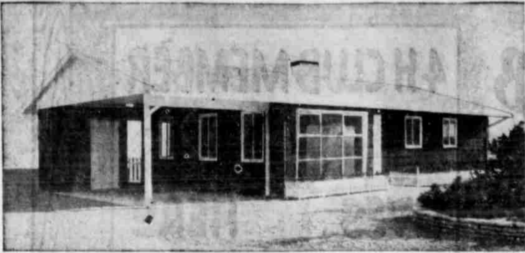
GLOBULAR HOUSE to start soon on an around-the-world tour to show how the average American worker lives. Tokyo, Japan will be the first stop. Then it goes to New Delhi, India. This dwelling made by United States Steel Homes, Inc., at New Albany, Ind., the housing subsidiary of U. S. Steel Corp., has been inspected by thousands, including President Eisenhower. He visited the home at the People's Capitalism exhibit in Washington, D. C. The entire exhibit, which is going on a global tour, is sponsored by the Advertising Council and the United States Information Agency of the State Department.
