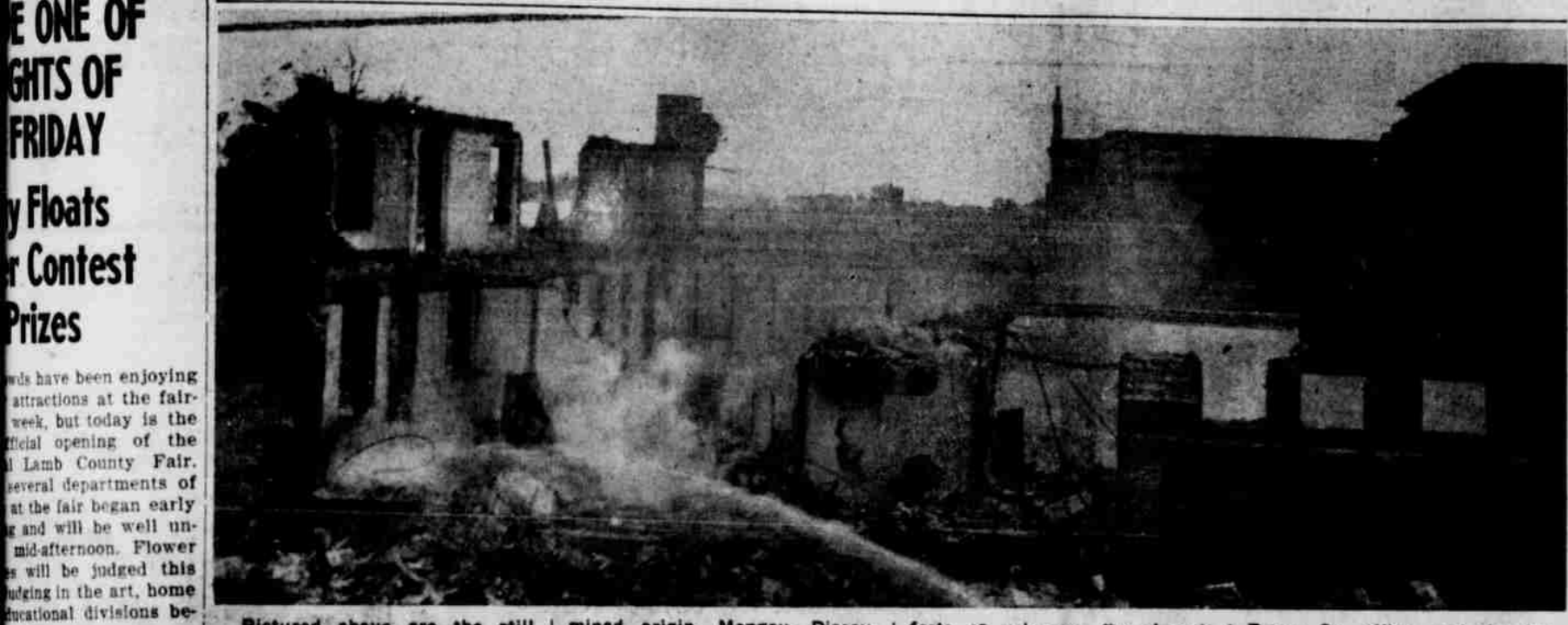
Pictured above are the still smoldering ruins of the Amherst hotel building, first brick structure in the city. The hotel and adjoining stores were razed by an early morning fire of undetermined origin, Monday. Discovered at 4 a.m. by Ross Hanks, the vacationing owner's brother, the fire already had a death grip on one section of the block in spite of efforts of volunteer fire departments from Amherst, Earth, Littlefield, and Sudan. Destroyed were the hotel, the drug store, Homer's barber shop, the school tax collector's office, Halsell Farms Co. office, and the Amherst Insurance Co. The ruins were still smoldering at 1 p.m. when this photo was taken.
