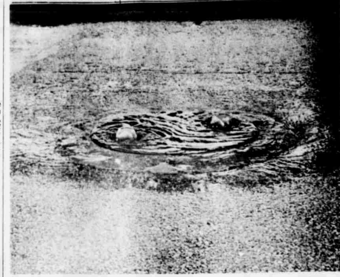
RAIN OVERFLOWS MANHOLE -- Following over 13 hours of rain this manhole located near Laguna Park was full and overflowing as the above picture shows. Rainfall in and around Littlefield measured from over two inches to almost four inches. Rain began falling Monday evening and continued until early afternoon Tuesday.
