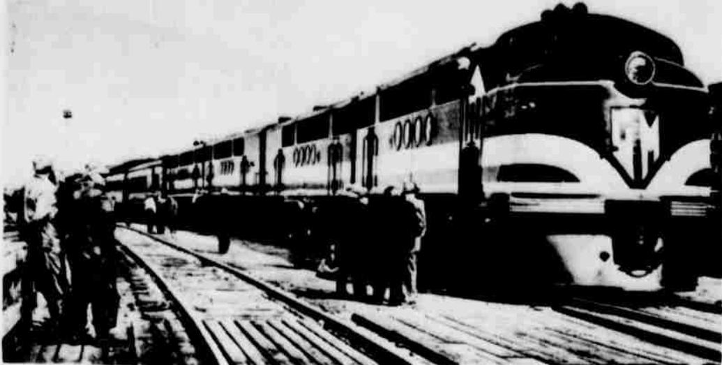
LA GRANGE, Ill. — Nation's first Diesel-powered, mainline freight locomotive, General Motors No. 103, is shown on tour after leaving the Electro-Motive Division plant here on the morning of November 25, 1939, to begin an 11-month, 83,000-mile test run over twenty Class I railroads. Number 103 demonstrated conclusively the superiority of Diesel over steam in hauling heavy ton-nages over the toughest grades under all sorts of operating conditions and became known as the "Diesel that did it" in the subsequent replacement of steam power by U.S. and overseas railroads. (Milwaukee Journal Photo.)
