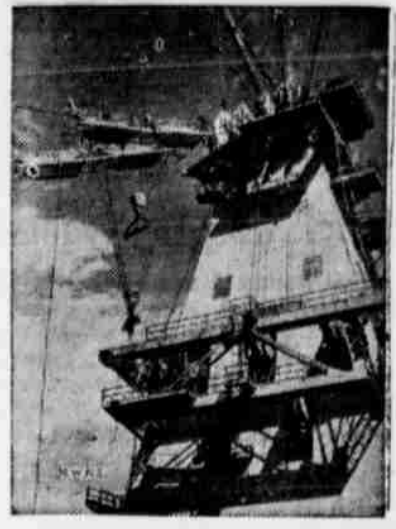
Apex of 460-foot tower built at the Shasta dam on the Sacramento river, California, to aid in the building of the largest concrete dam in the world, with the exception of Boulder. The dam will conserve the water of the Sacramento river for irrigation and power.
