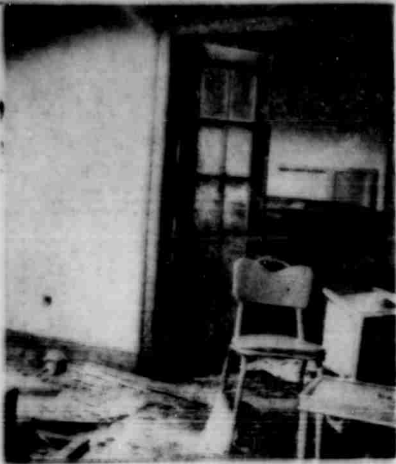
THE INSIDE of the Avery home is shown here just before it started to rain Monday morning. The walls of the house were still in good shape but the furniture is badly misplaced.
