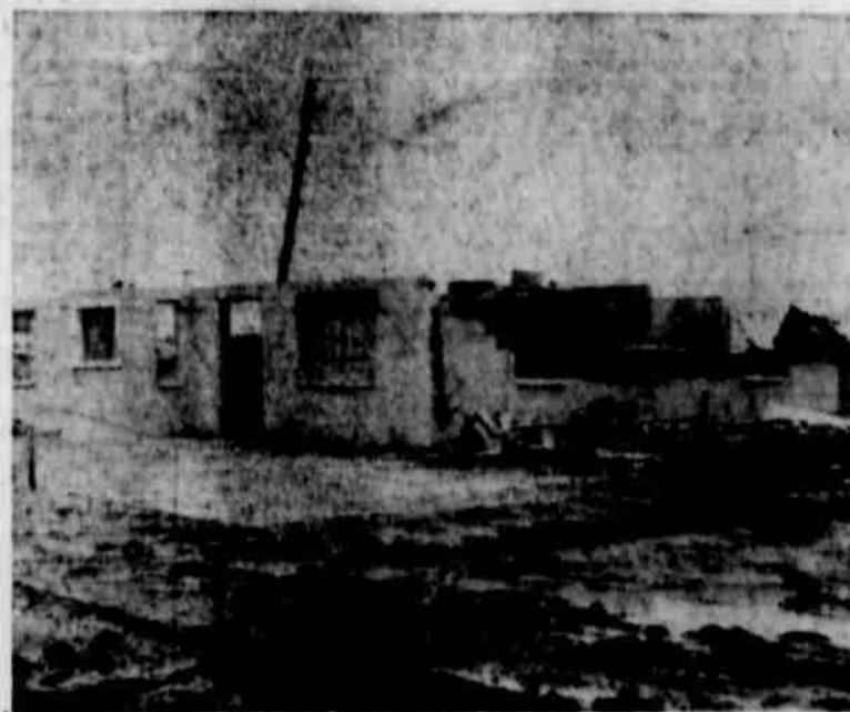
ONLY THE WALLS remained of this concrete block building which served as the office building for the Hart Camp Co-op Gin. All of the gin property in the locale was a complete loss.
