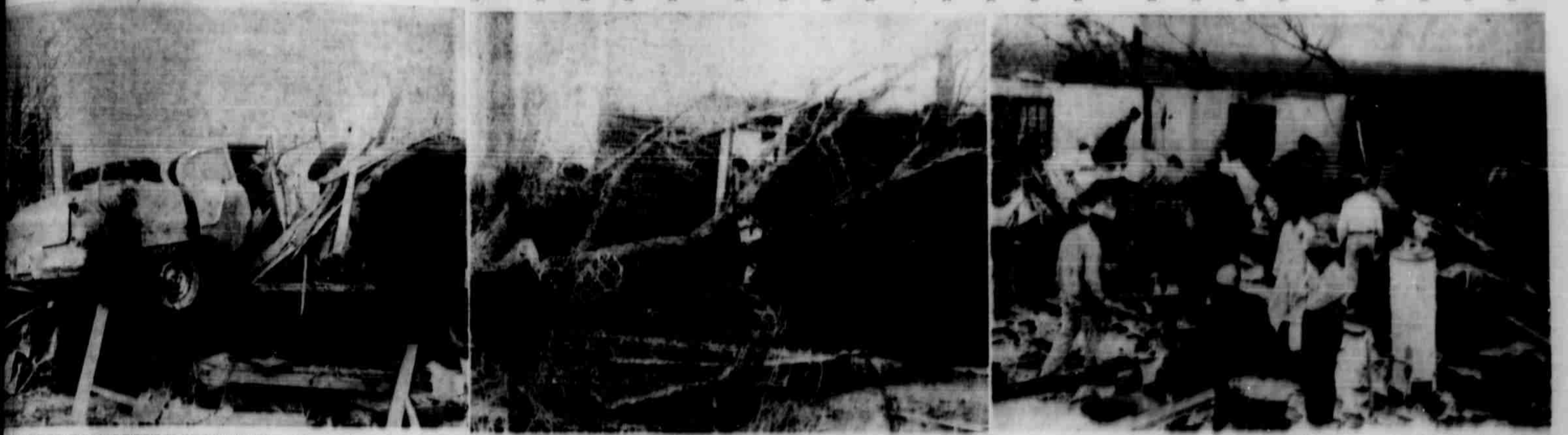
PADON HOME COMPLETELY DESTROYED — Shown above are scenes showing all that is left of the J. E. Padon home southwest of Spade after the tornado struck there Sunday night. In the first picture the 1954 Oldsmobile that was lifted from the garage and landed on top pinning Mrs. W. N. Yant, mother of Mrs. Padon, underneath
