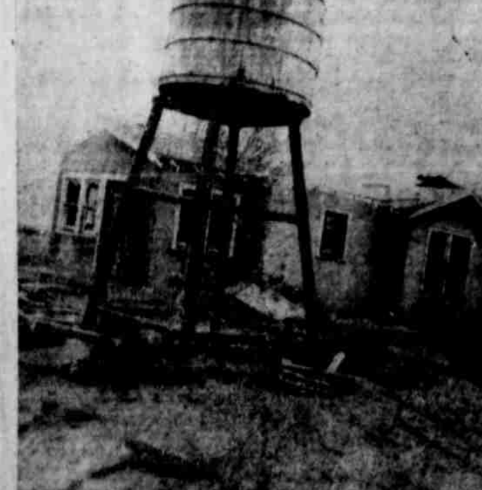
ROBERT AVERY'S HOME one mile south of Whitharral is shown here with the roof completely gone and the surroundings in shambles. His windmill was blown away but the water tank is shown still standing and in good condition.
