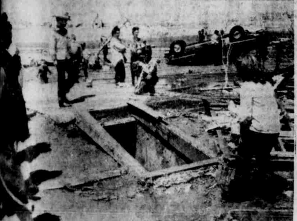
STORM CELLAR saved the lives of members of the Ben Waters family northwest Whitharral, during last Sunday's tornado. Here is shown the door of the cellar near the entrance. The automobile shown in the background was blown about 100 yards while in flight tore the door from the hinges, tearing a small part of the top of the storm cellar off. Three houses were destroyed within a radius of half a mile. All furniture and clothing, were lost by members of the families. (Staff Photo)
