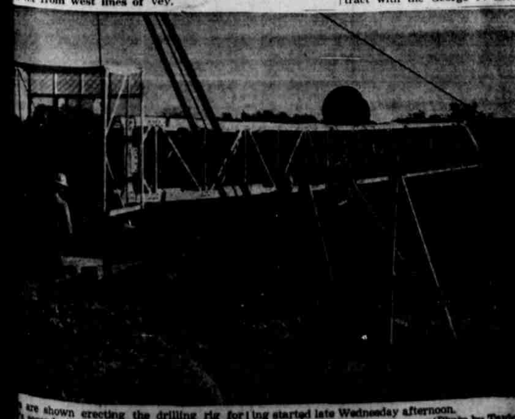
are shown erecting the drilling rig for ing started late Wednesday afternoon. second oil well, in the city park. Drilling (Photo by Taylor)
