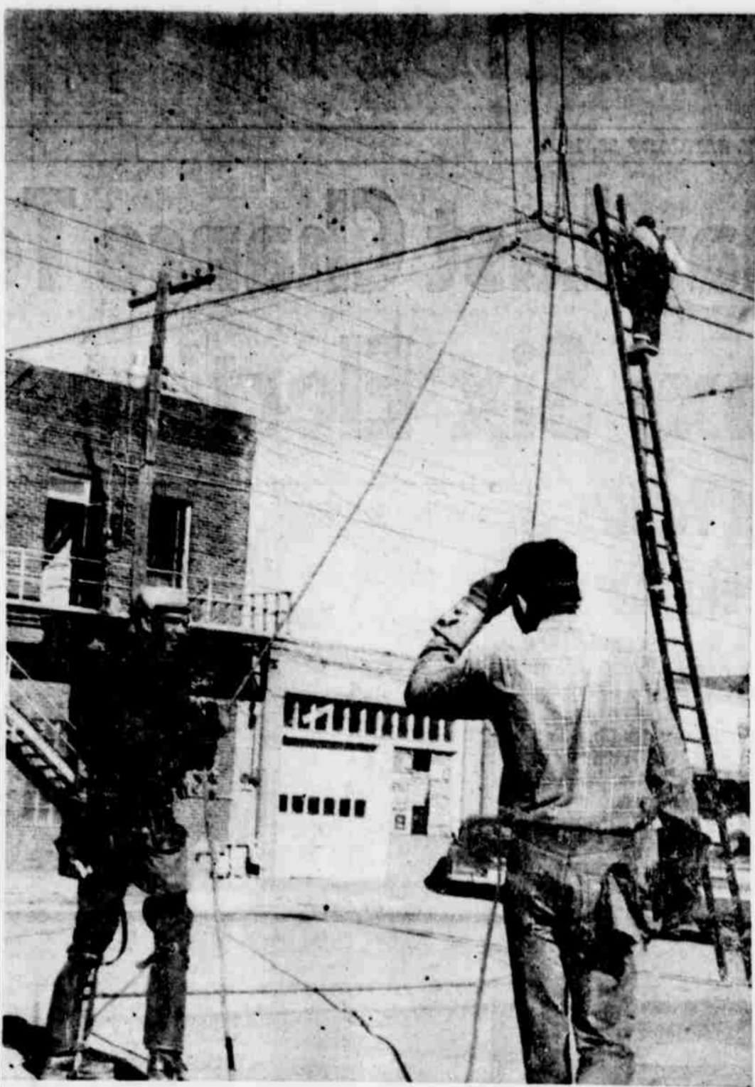
CONNECTING THE OLD WITH THE NEW! General Telephone workers this week are connecting the old system with the new. They are shown putting up connecting cable to the company's new plant at 5th and Twitchell. Plans call for the phone system to be converted to dial June 1.
