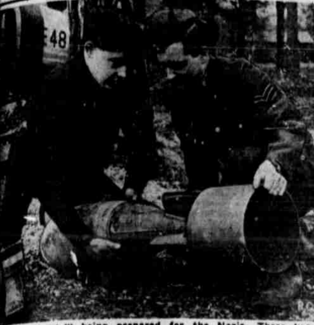
"Bundle of grief" being prepared for the Nazis. These two mechanics have fused this bomb and are securing the tail fin in its proper position. Then they will load the sensitive "egg" under the wing of the vicious "Hurry-bomber" behind.
