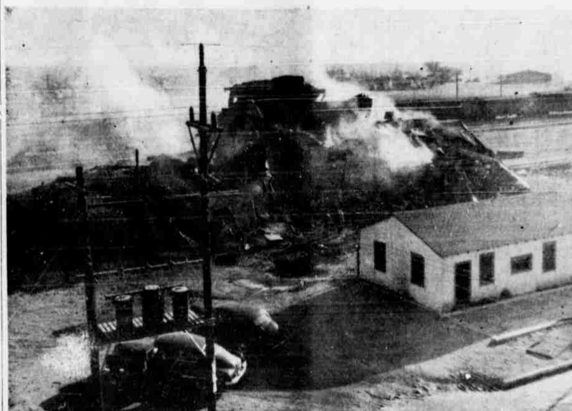
BLAZE LEAVES WALKER ELEVATOR —A $115,000 fire which destroyed the P. W. Walker Grain and Seed Company elevator here last Wednesday was caused by an electric motor in the top of the elevator, Walker said. The three-hour fire leveled the 180-foot sheet metal building and ruined 4,000 bushels of wheat and 2,300,000 pounds of grain sorgums. Walker said Tuesday that he has not made any plans for re-building the elevator. He added that the damaged grain had been sold to a Mr. Moore in Justin, Texas, and that he had no idea what Moore plans to do with the grain. (Photo By Taylor's Studio)
