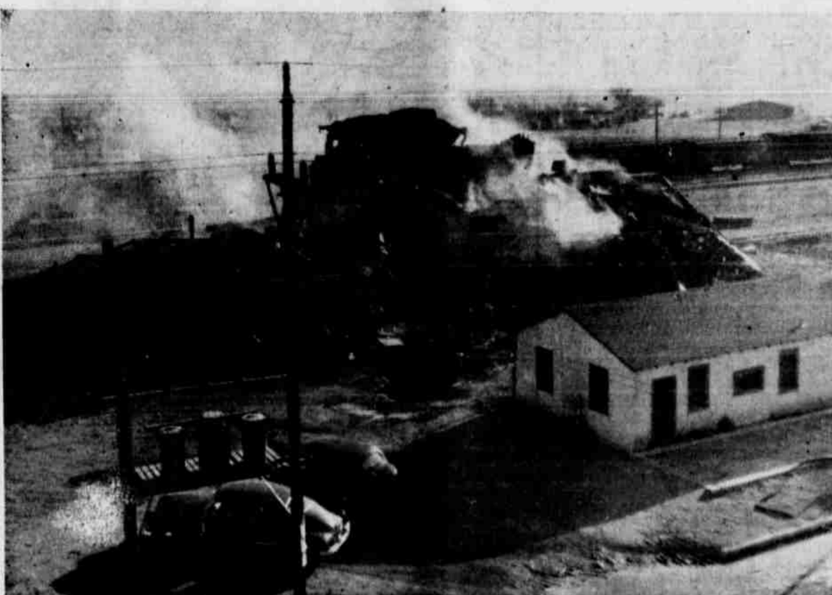
BLAZE LEAVES WALKER ELEVATOR—A $115,000 fire which destroyed the P. W. Walker Grain and Seed Company elevator here last Wednesday was caused by an electric motor in the top of the elevator, Walker said. The three-hour fire leveled the 180-foot sheet metal building and ruined 4,000 bushels of wheat and 2,300,000 pounds of grain sorghums. Walker said Tuesday that he has not made any plans for re-building the elevator. He added that the damaged grain had been sold to a Mr. Moore in Justin, Texas, and that he had no idea what Moore plans to do with the grain. (Photo by Taylor's Studio)
