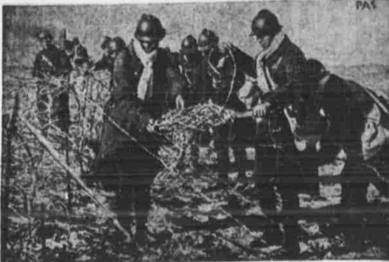
TUNIS, Tunisia... A detachment of soldiers string barbed wire before one of the new fortifications in the Mareth Line. The wire is strung on spikes which have been imbedded in blocks of concrete and buried in the ground.
