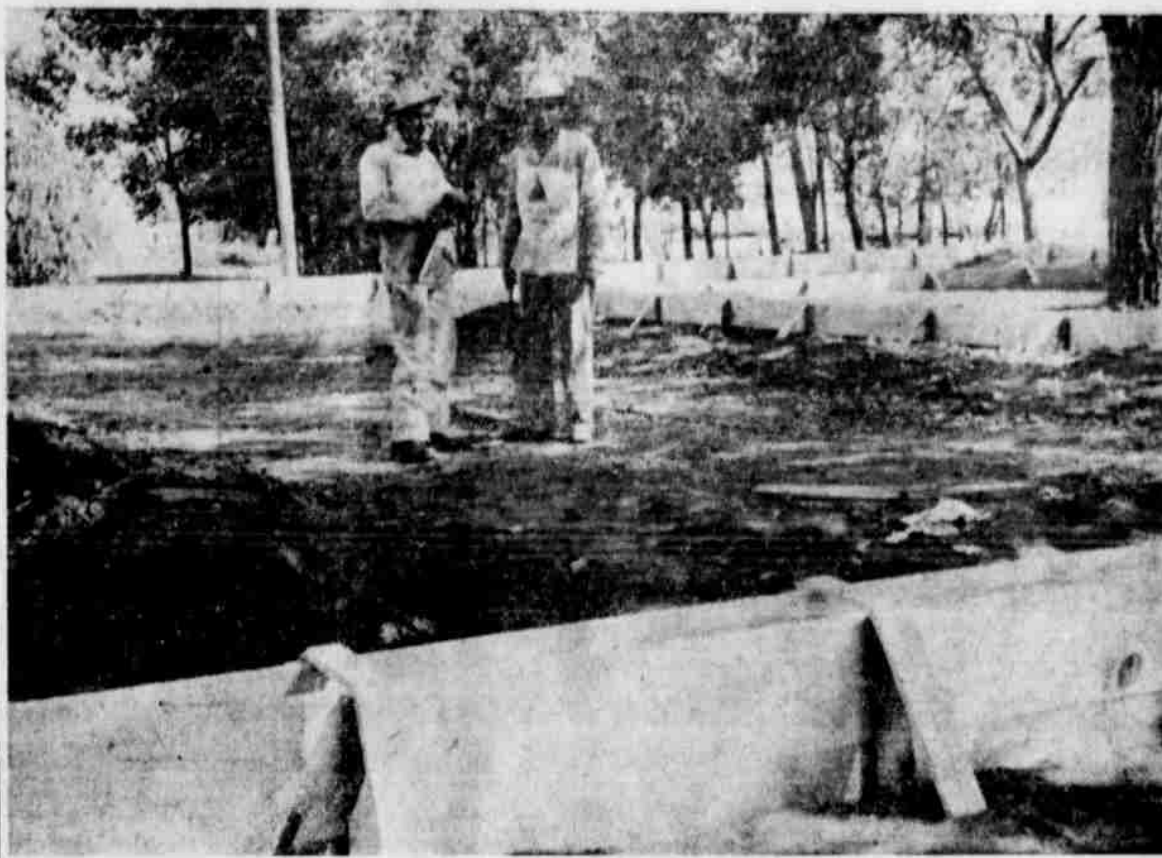
Construction of the Sudan Community building got underway here last week when forms were laid for the foundation. The contract to build the building was let to Higginbotham Bartlett Lumber Company of Sudan. Carpenters pictured above who are working on the construction are Harlon Reese and Cecil Testerman. (Scott Photo)
