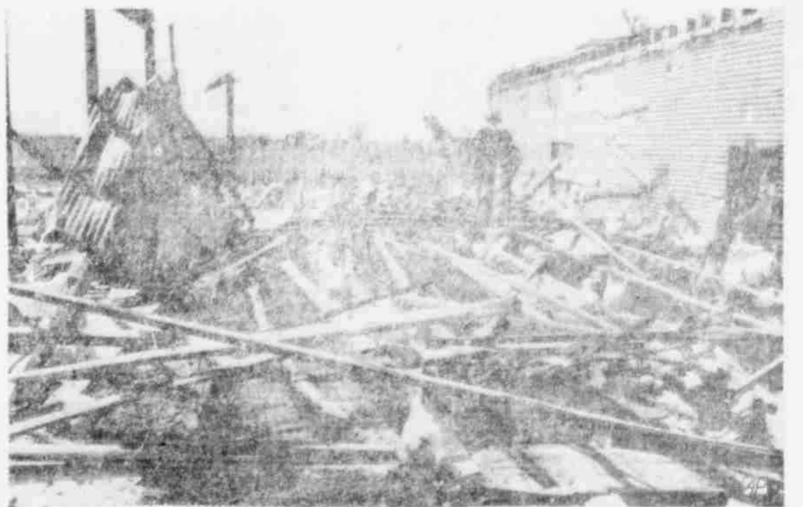
Chickens which survived a storm which struck the W. B. Harrison chicken ranch a mile west of Stamford, Tex., run wildly amid the wreckage of one of the main buildings. Several hundred chickens were killed. Three unidentified men survey the damage, estimated at $15,000. (AP Wirephoto)
