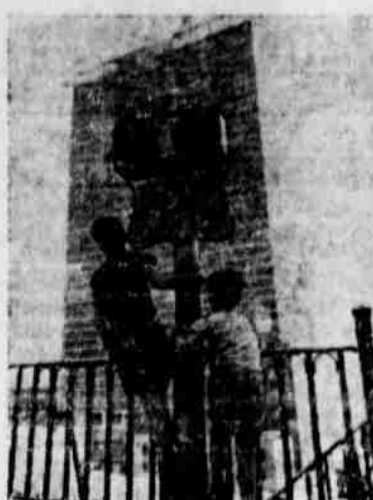
MONUMENT TO THEIR FUTURE — Two young Americans from New York's East Side stand under a 'dead end' sign and gaze hopefully toward the uncompleted United Nations headquarters building.
