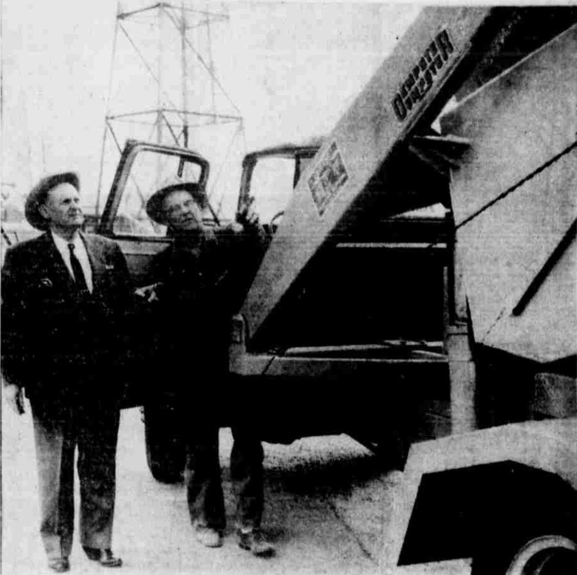
IT WON'T BE LONG NOW—Mayor Ellis Foust, left, and City Commissioner Bob Cox look over the new truck which will be used to run the Dempster-Dumpster system here. Installation of the system should be complete by Nov. 1. Sid Patten, representative of the system, is scheduled to arrive here Monday to begin installation of the trash removal system. Almost 30 containers which will be placed throughout the business district are scheduled to arrive this week. Plans for the installation will be discussed tonight at a regular city commission meeting. (STAFF PHOTO)
