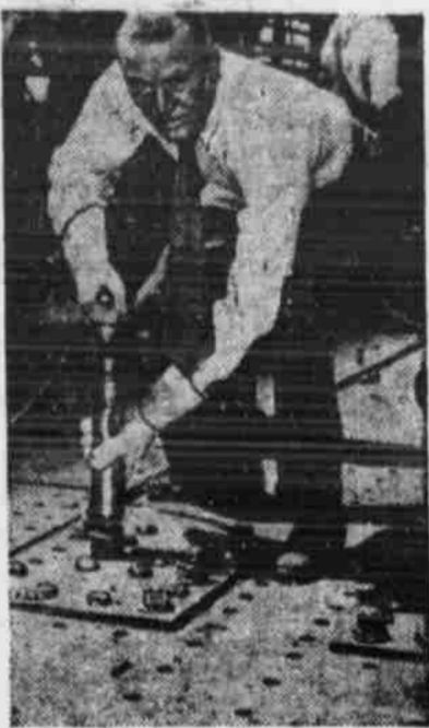
NEWPORT NEWS, Va. . . . Rear Admiral E. S. Land, chairman of the United States Maritime Commission, driving the first rivet in the keel of a new liner which is to be the largest and fastest ever constructed in this country. When completed, this vessel will replace the old Leviathan in the transatlantic trade.
