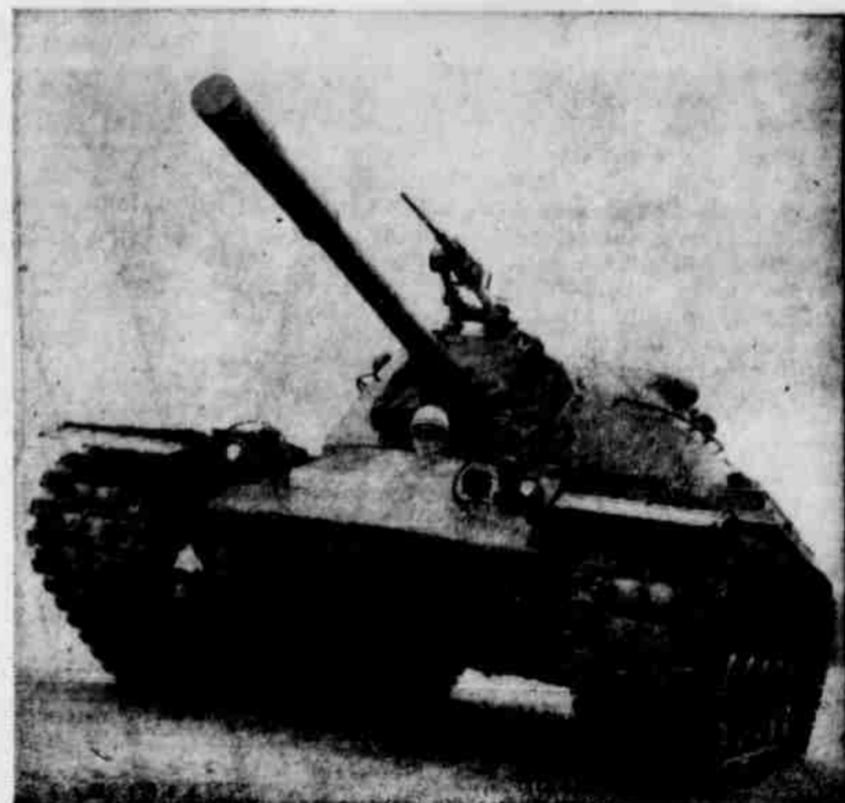
This is the Army's newest Tank, the Patton 48, described as the most modern medium tank ever made for our troops. The new combat vehicle has just been unveiled at the Chrysler Delaware Tank Plant where it was built. Design of the tank was completed by Chrysler Corporation to specifications of Army Ordnance. Extreme maneuverability of the Patton 48—its low silhouette—one piece cast armor hull and improved firepower all combine to make the Patton 48 a formidable fighting machine.
