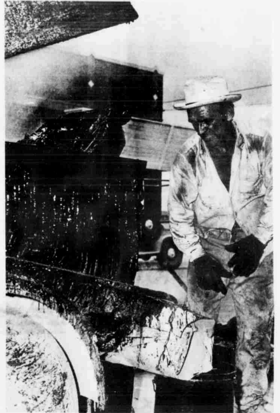
A HOT JOB on a hot day! With sweat pouring down his face, Don Wallace of Tracy Perkins Roofing Co. checks the temperature gauge on the tar pot. He constantly reads 450 degrees, whether the weather is 97 degrees—as it was when the camera caught him at work Friday afternoon—or whether it's near zero.
