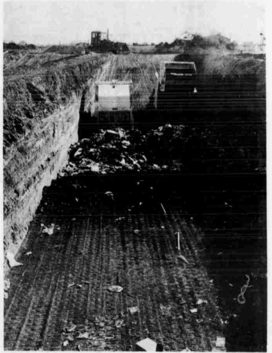
MOUNTAINS OF GARBAGE are buried daily at the city dump ground since the state ordinance forbidding burning went into effect in July, 1969. In the foreground are the two city collection trucks making their dump at the end of a day, and the caterpillar operator is waiting to move in and bulldoze the garbage under. Last year 36,020 tons of garbage was buried at the city dumping site.
