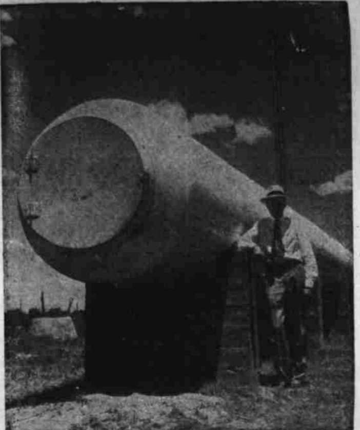
Butane Storage —This giant storage tank—56 feet, one inch in length and with a capacity of 6,000 gallons—has been added to the facilities of Fraley & Co., Butane dealer, for serving this area with Butane gas. Beside the tank is new assistant manager for the company, Marvin Imken, who has offices in Abilene. Fraley & Co. serves the West Texas area from Abilene, Big Spring and Graham.
