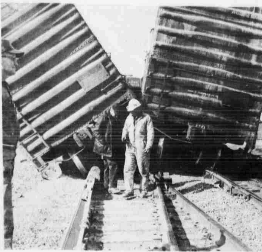
STRONG WINDS blew these two railroad cars together early Tuesday afternoon at the Nipak spur. The car on the left was empty and the one on the right was loaded with chemicals to be left at Nipak. Looking at the twisted left rail are E. D. Perdue, brakeman, extreme left foreground; Mark Etter, conductor; and A. V. McGowan, track supervisor. Workers were switching cars when they noticed the cars rolling toward each other.
