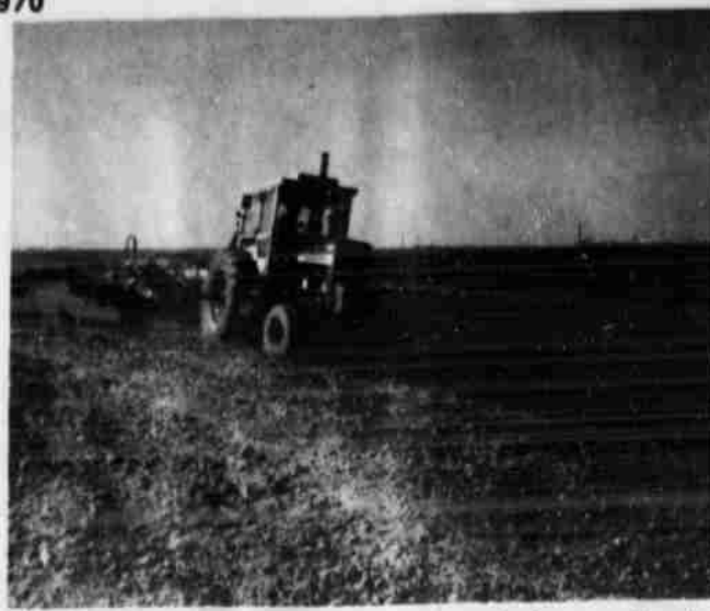
DIVISION AND parallel terraces are being constructed on the K. E. Priboth farm, three and one-half miles south of Littlefield. This is a double belt terracing machine used in building the terraces as part of conservation measures through the Lamb County ASCS and SCS offices.
