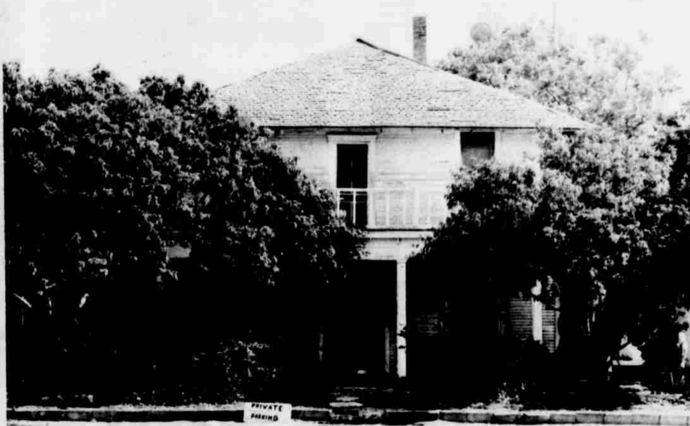
THE OLD SMITH HOTEL is one of Littlefield's oldest landmarks, and Mrs. Lorado McKnight has lived in the hotel most of the 57 years it has been in Littlefield. First erected on Delano Avenue in 1913, the hotel was moved to its present site on Fourth Street in 1923.
