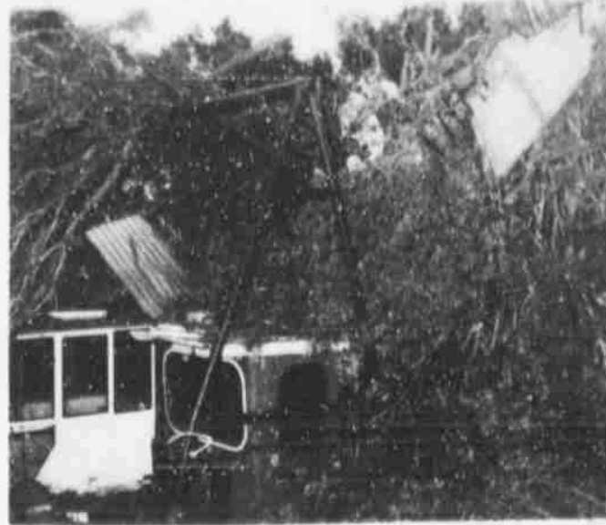
A BARN ROOF was lifted approximately 14 feet into the air and driven into these elm trees at the T.C. Faver farm Friday evening. The top portion of the trees were broken and twisted off but protected these tractor cabs.
