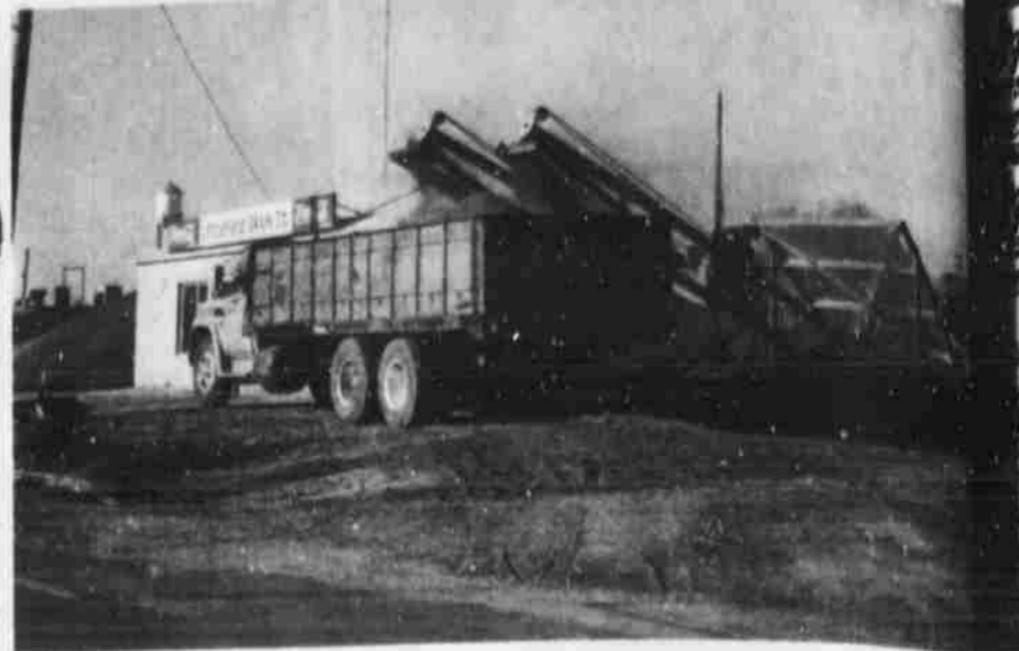
CLEANUP PROCESSES were nearing completion by presstime Wednesday. Littlefield Grain Co. According to Doyle Dean, owner of the elevator which burned 18, approximately two-thirds of the grain will be salvaged. Front loaders picked grain and dumped it through a huge screen. The screened grain was re-screened it was loaded on trucks.
