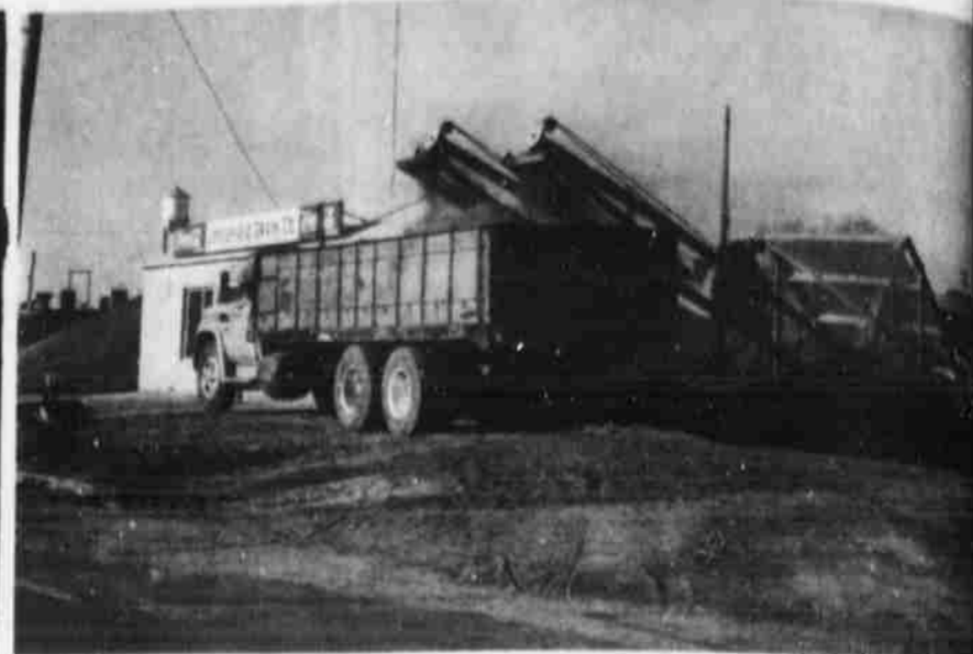
CLEANUP PROCESSES were nearing completion by presstime Wednesday. Littlefield Grain Co. According to Doyle Dean, owner of the elevator which burned 18, approximately two-thirds of the grain will be salvaged. Front loaders picked grain and dumped it through a huge screen. The screened grain was re-screened and it was loaded on trucks.
