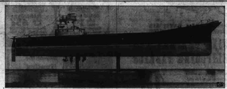
SOMETHING NEW IN NAVAL NEWS\_A pro of the Sea Otter (shown in model), a new type inexpensive cargo ship which, says the U.S. navy, might challenge the subma ship, capable of 12 knots, is 270 feet long overall and can carry a net 1,500 tons of cargo. No fewer than 16 gasoline engines su in motor boats drive the vertical shaft. Ship's flat silhouette would make it a poor target for hostile surface vessels or airo
