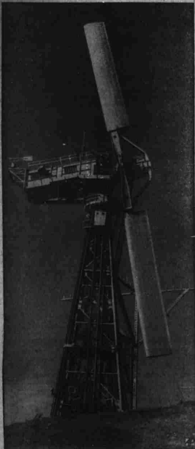
DOING A GOOD TURN —An 18-mile-an-hour wind is needed to turn the 175-foot blades of this new windmill electric generator atop Grandpa's Knob at Hubbardton, Vt., which, builders estimate, should generate enough current to supply 2,000 homes with its 1,000 kilowatts at 2,400 volts. Its position on a peak 2,699 feet above sea level promises constant wind.
