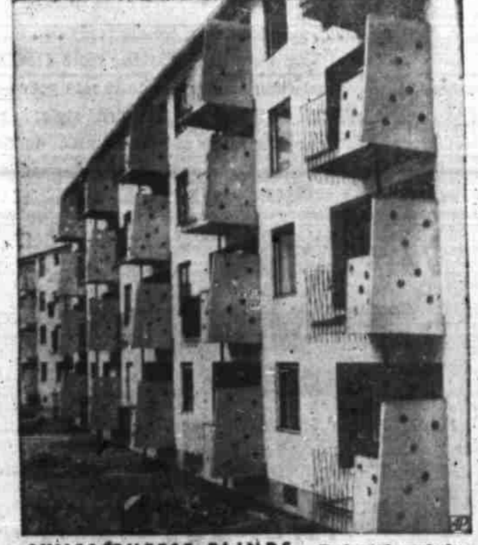
SWISS CHEESE BLINDS — Perforated sunshades are conspicuous on balconies of new apartment houses in the U. S. sector of West Berlin. Holes permit limited vision.
